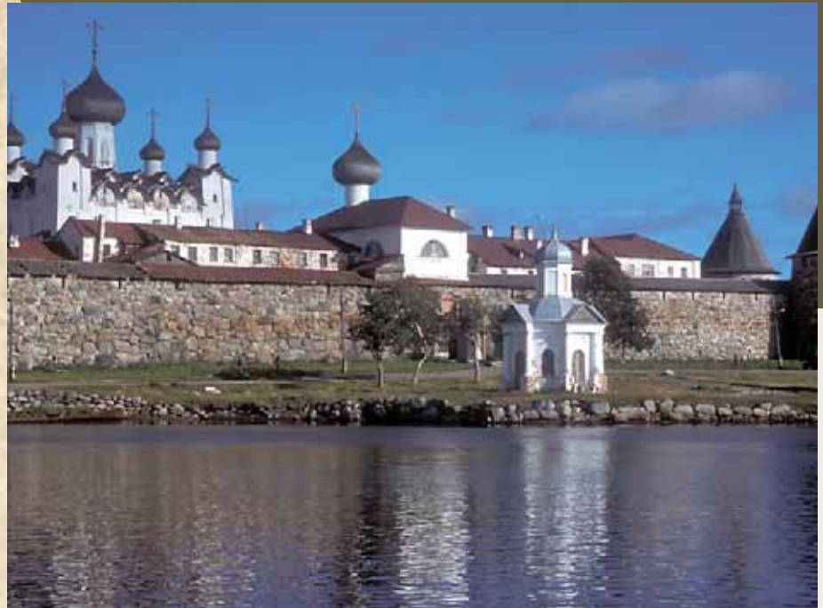
Solovetsky's six-meter-thick kremlin walls were built from the island's rock
