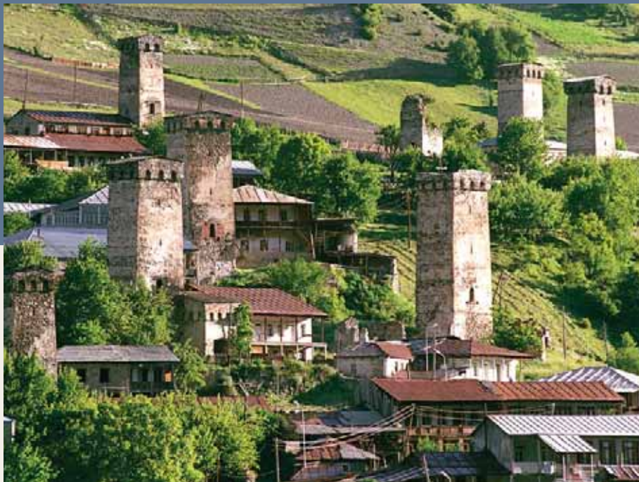
Tower architecture of Svaneti, Georgia
